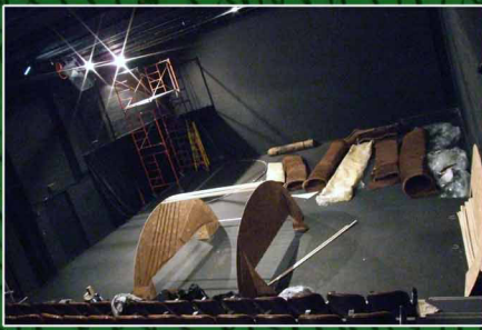
Building the form
